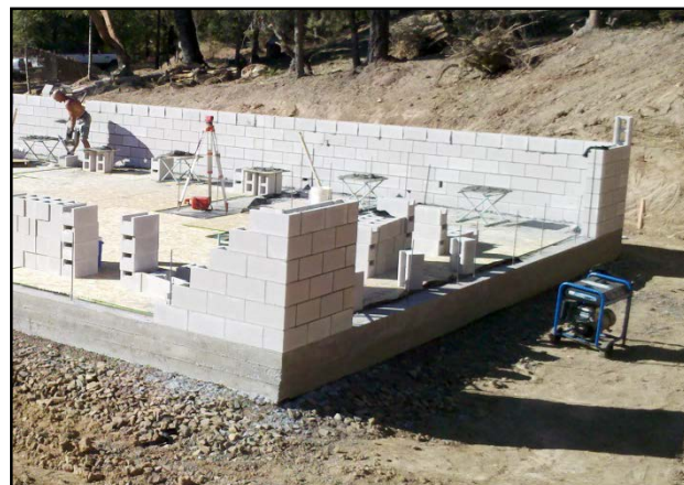
Figure 2: Photograph of a lead section of block wall.
